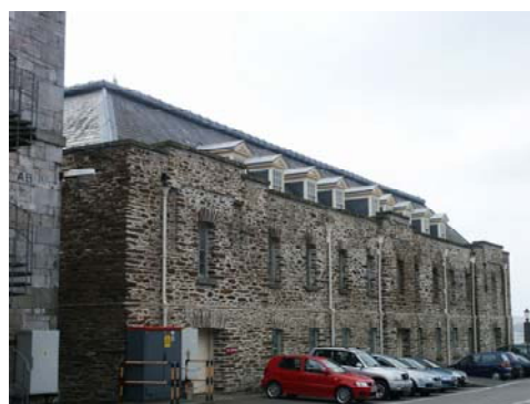
Storehouse No 4, Morice Yard (Grade II*) (Photograph by Jess Maslen)
